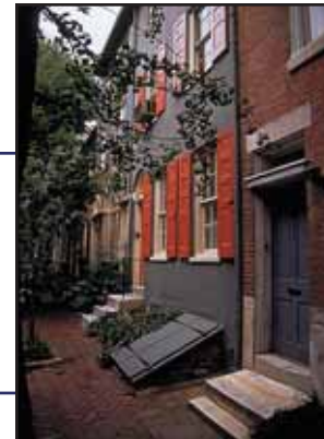
Raised stoop entrance for multiple apartments
