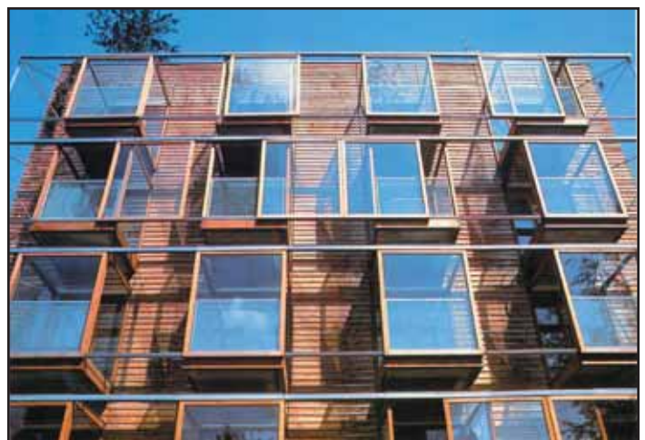
Creative articulation of windows and façades
